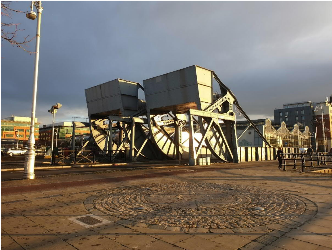
Existing George's Dock Scherzer's bridge to be relocated– looking from the River Liffey
